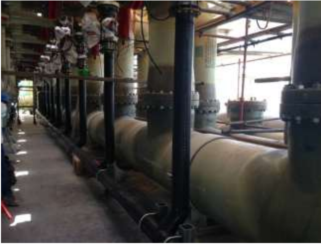
HDPE PIPE INSTALLATION IN MARAFIQ
